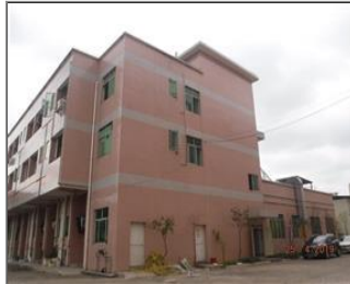
External photo(s) of the production unit(s) Dormitory building.JPG
